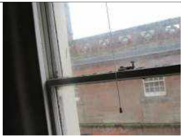
5.24 second floor window sashes
