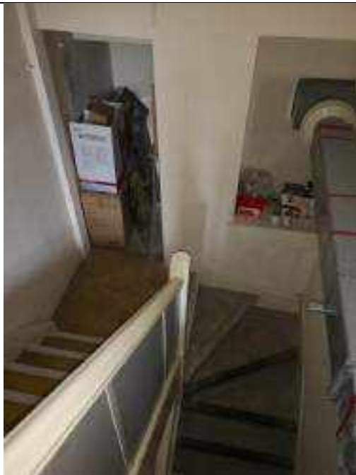
6.53 stair at second floor landing
