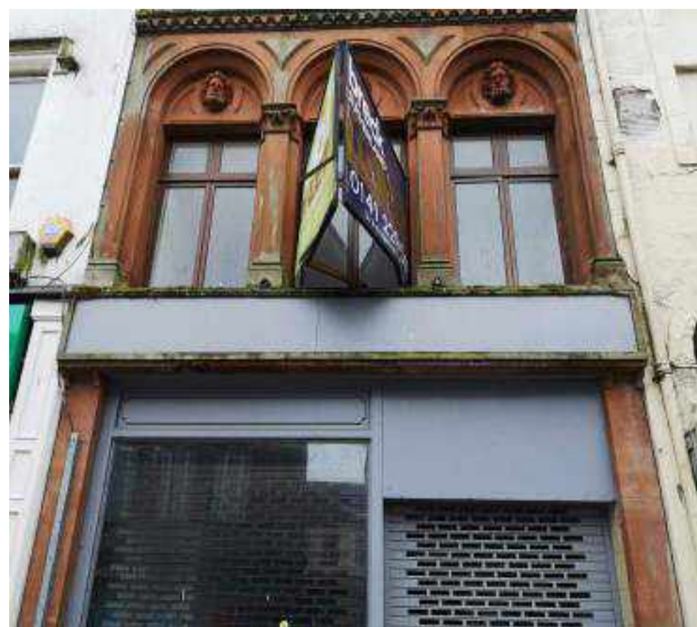
111 High Street Street view
