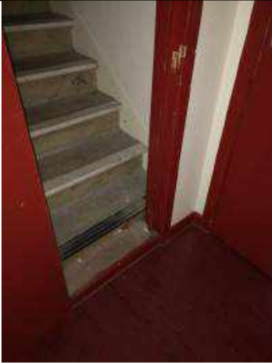
6.51 turning stair to second floor
