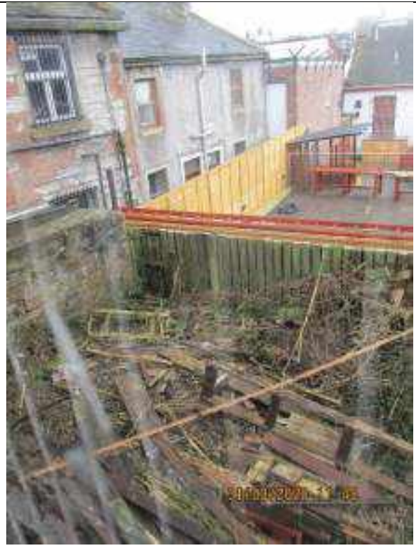
6.100 view of rear yard from window
