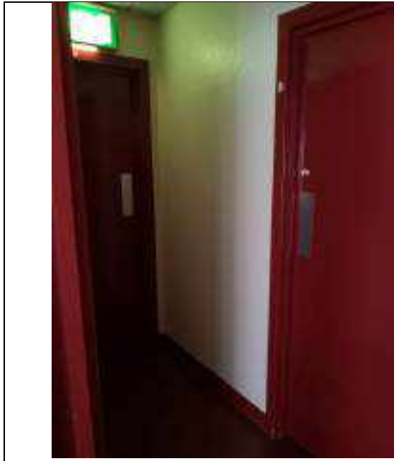
6.61 first floor doors
