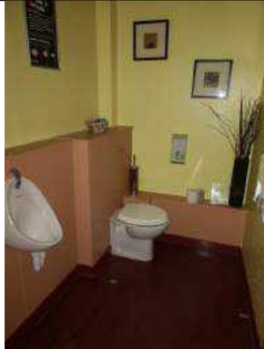
6.44 toilets pipe boxing
