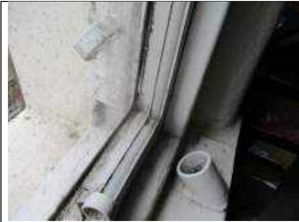
5.25 second floor window sill corner
