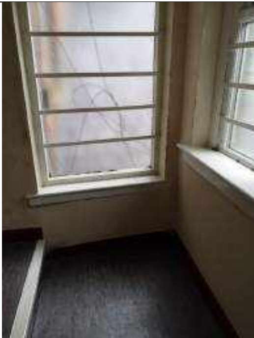
5.27 windows to rear cantilever
