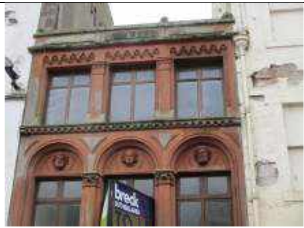
5.14 Stone façade to upper floors
