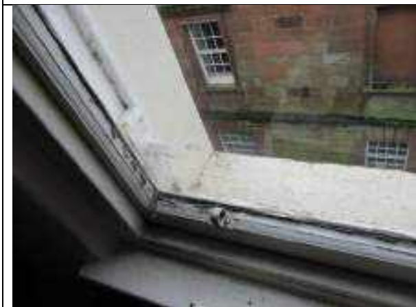
5.23 second floor window lower sash
