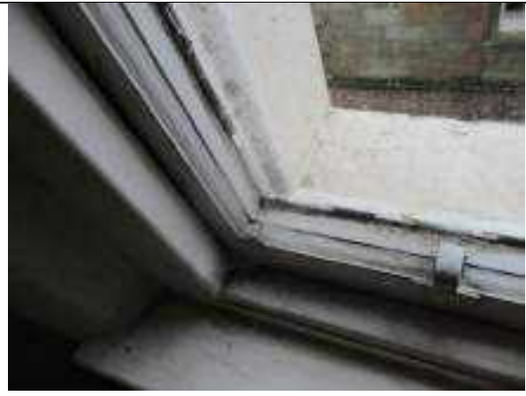
5.26 second floor window sill corner
