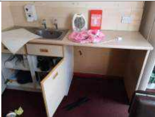
6.41 sink and worktop in kitchen
