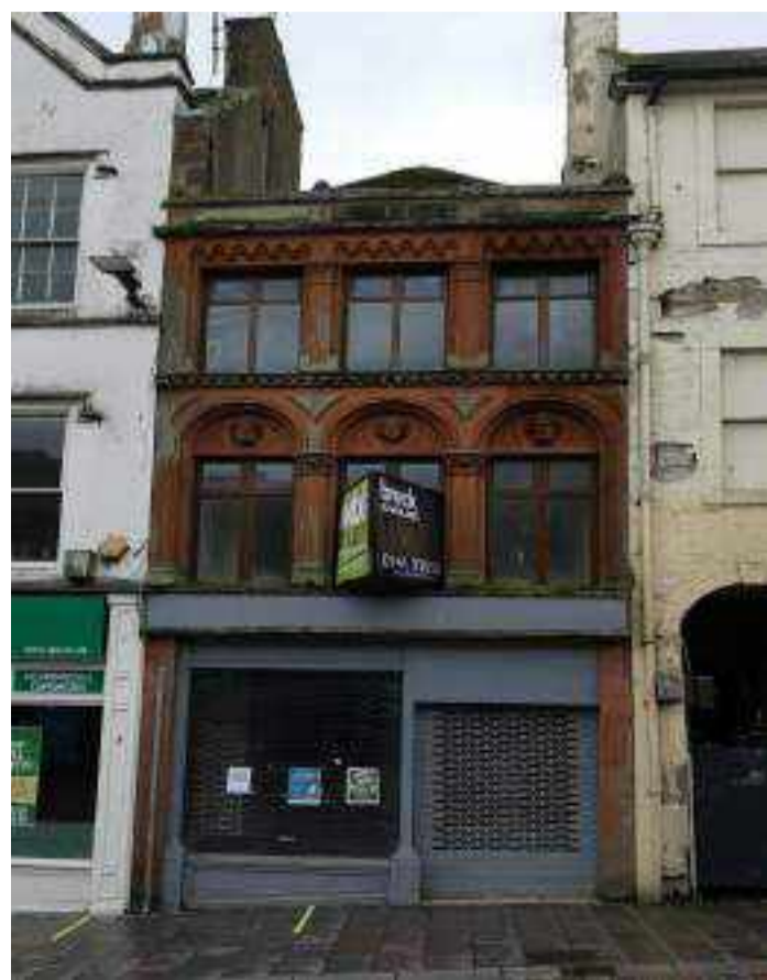
111 High Street Street view
