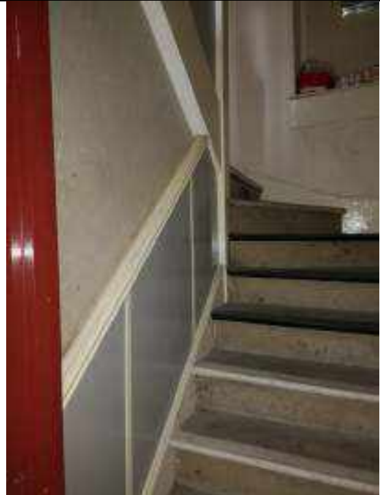
6.52 turning stair to second floor
