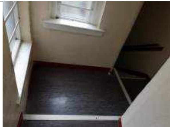
6.46 stair to first floor landing in cantilever projection
