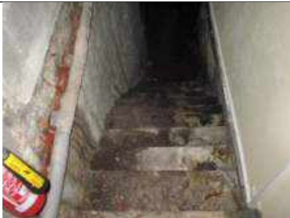
6.45 stairs to cellar
