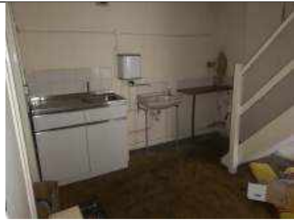
6.42 second floor rear right room sinks
