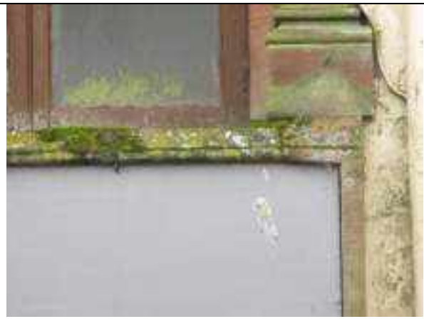
5.18 stone sill above shop front
